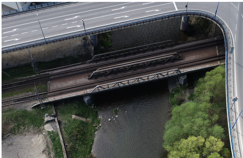
Figure 1 Case study railway bridge
