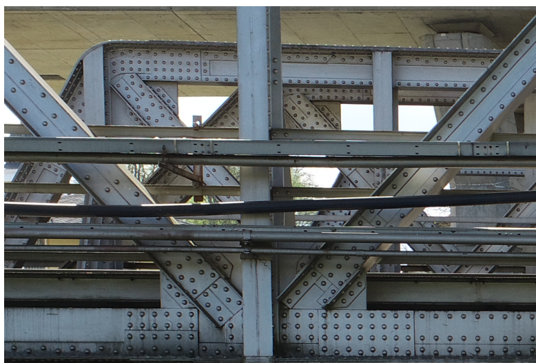
Figure 2 Detailed look of railway bridge construction
